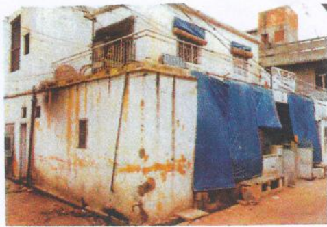
The old hospital building of the RMC (below) and the new one (bottom)
